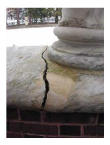
Part of the installation, but not related to the accident, the brickwork flanking the main entrance, is showing the same symptoms, and requires the same treatment, as the rest of the masonry that has been repointed over the past several decades.
